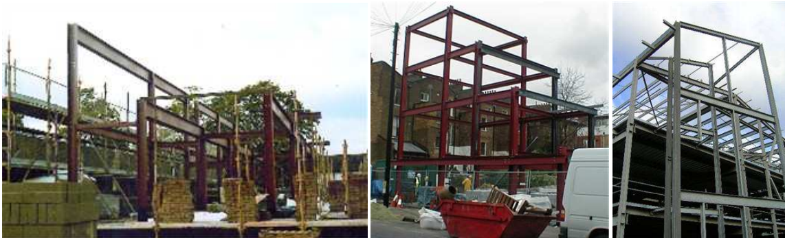
BedZED (Beddington Zero Energy Development) – BowZED à Londres – ( Source: © BioRegional ( www.bioregional-reclaimed.com ) )
